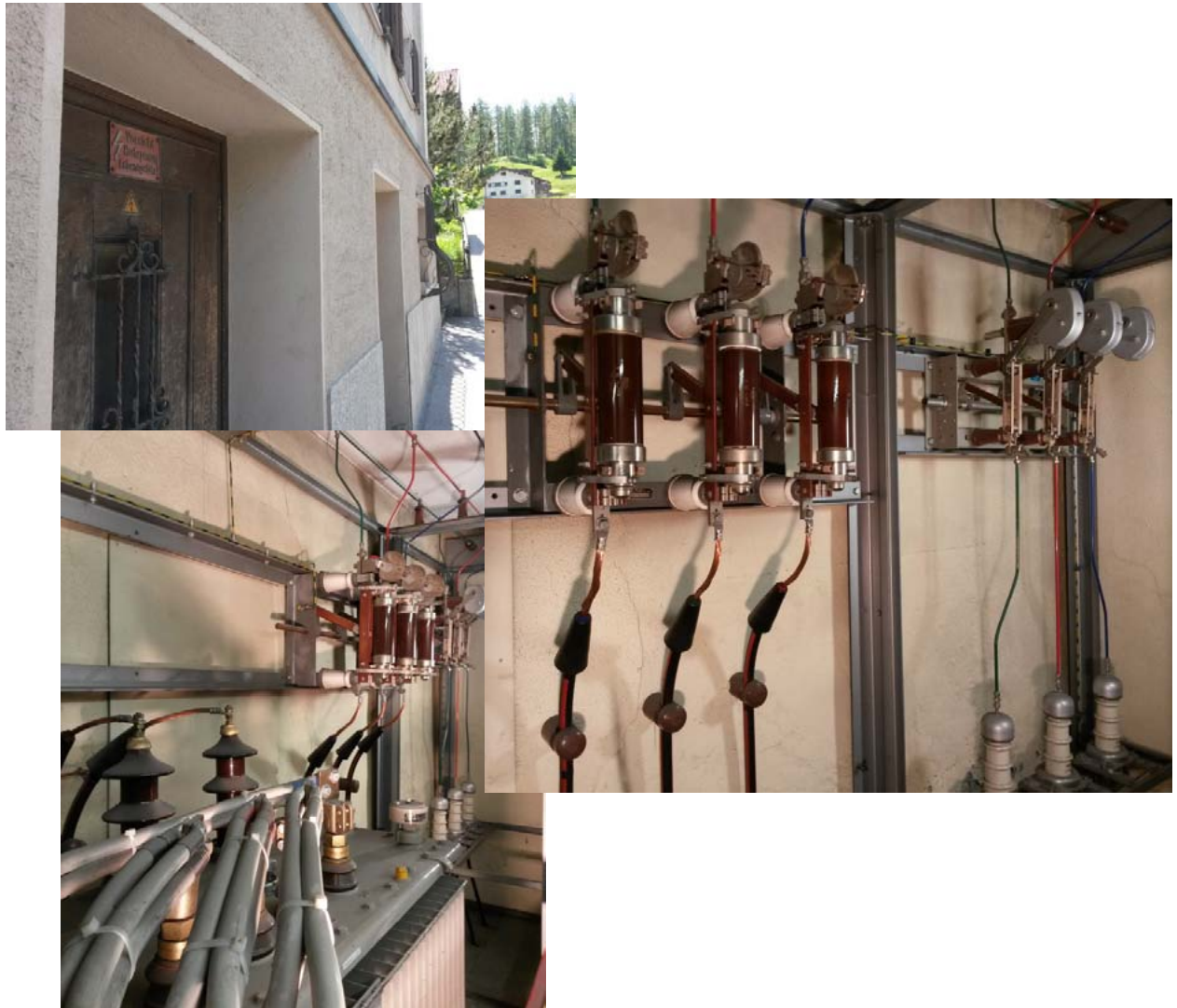
Alte Trafostation Krone in Churwalden
